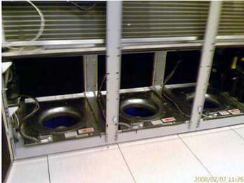
With the fans in the lower position, the BMS was allowed once again to bring the floor to an average static pressure of 0.011" w.c.. After a period of stabilization, the return air was measured at each unit and several supply air measurements were taken on perforated tiles. The air flow was recorded at a total of 33,112 CFM. The average static pressure on the floor was 0.010" w.c. and the fan speed with the fans in the lower position, dropped to 88% of their maximum.
